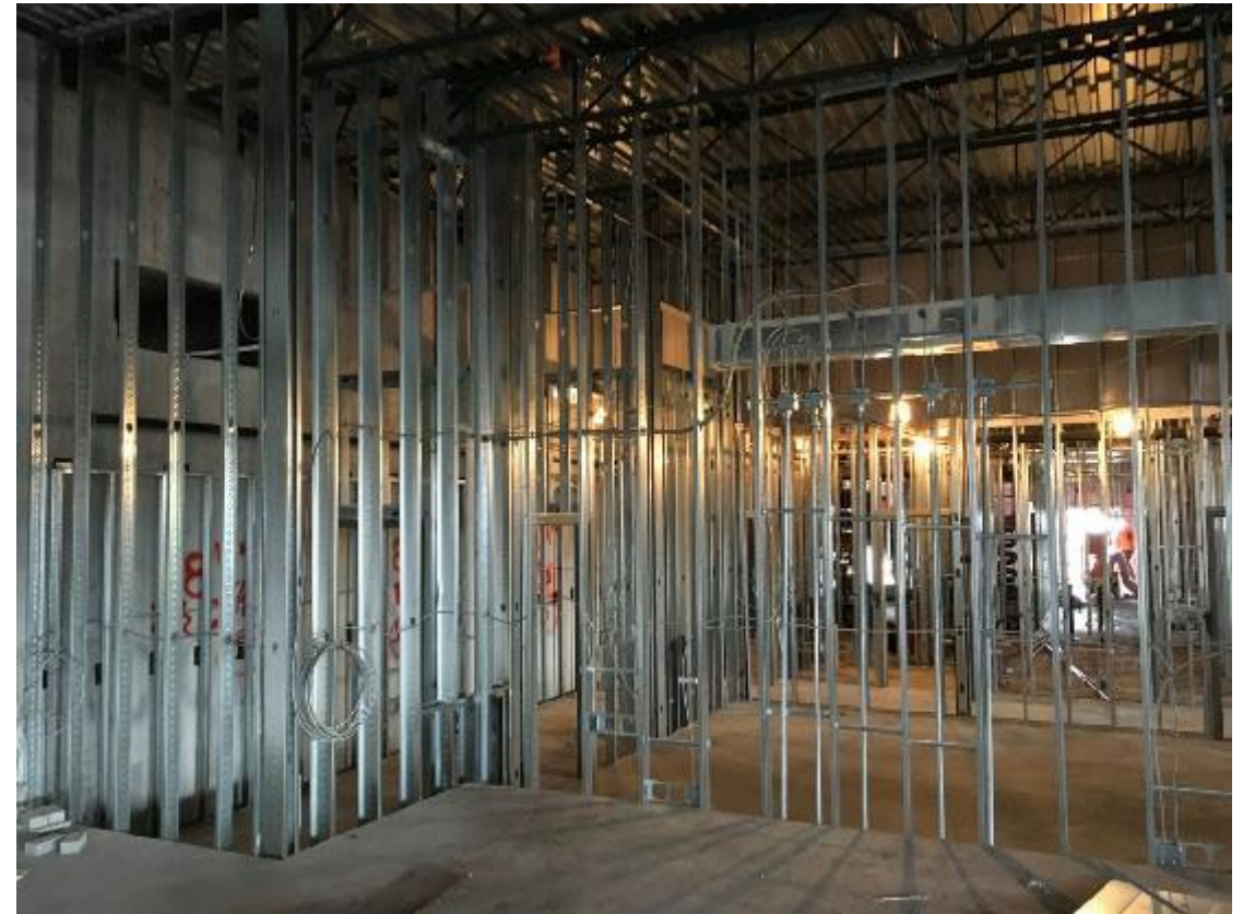
Interior Classroom Framing
