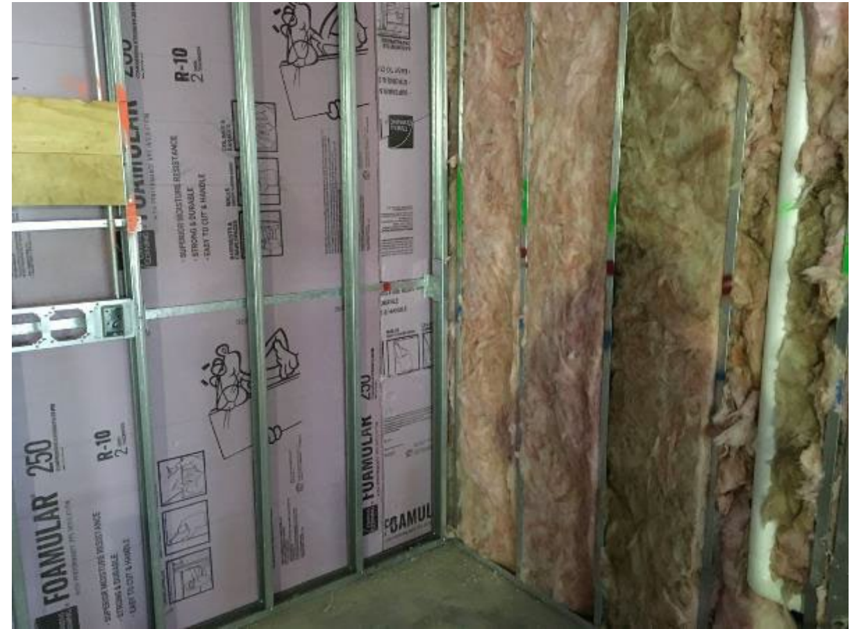
Interior Wall Insulation
