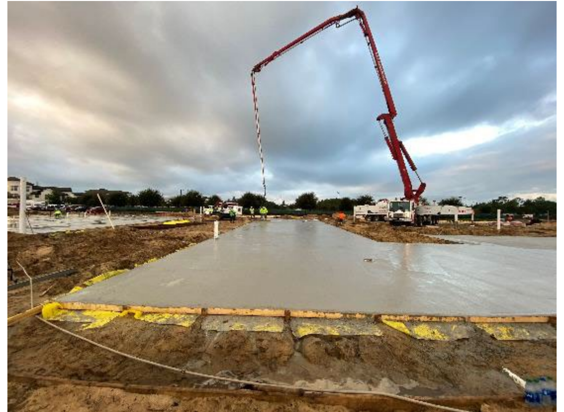
Pouring of Tilt Panels with a Boom Pump
