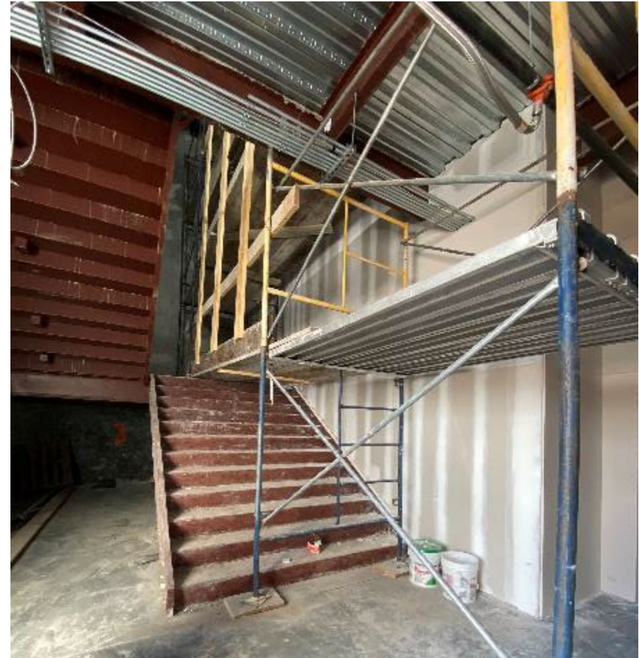
Interior Wall Finishing at Stairwell
