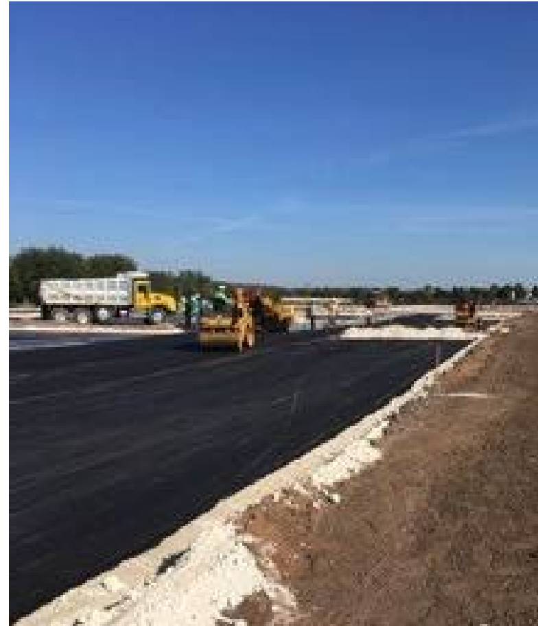
Asphalt paving for Parent Parking
