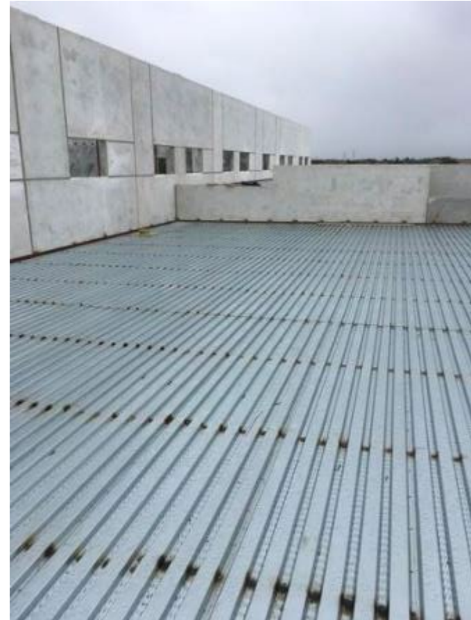
Roof Deck Installation
