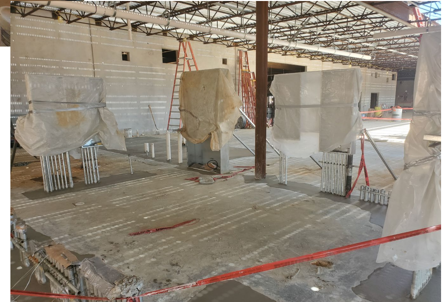
Below is rough in of Building 1 Electrical room
