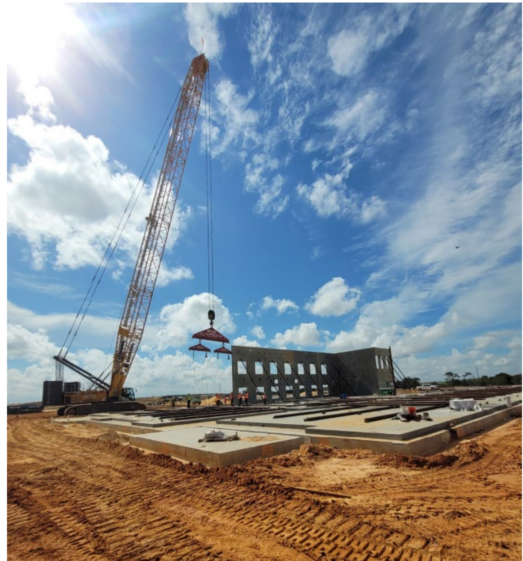
Above is erection of tilt panels at Building 5 looking SE
