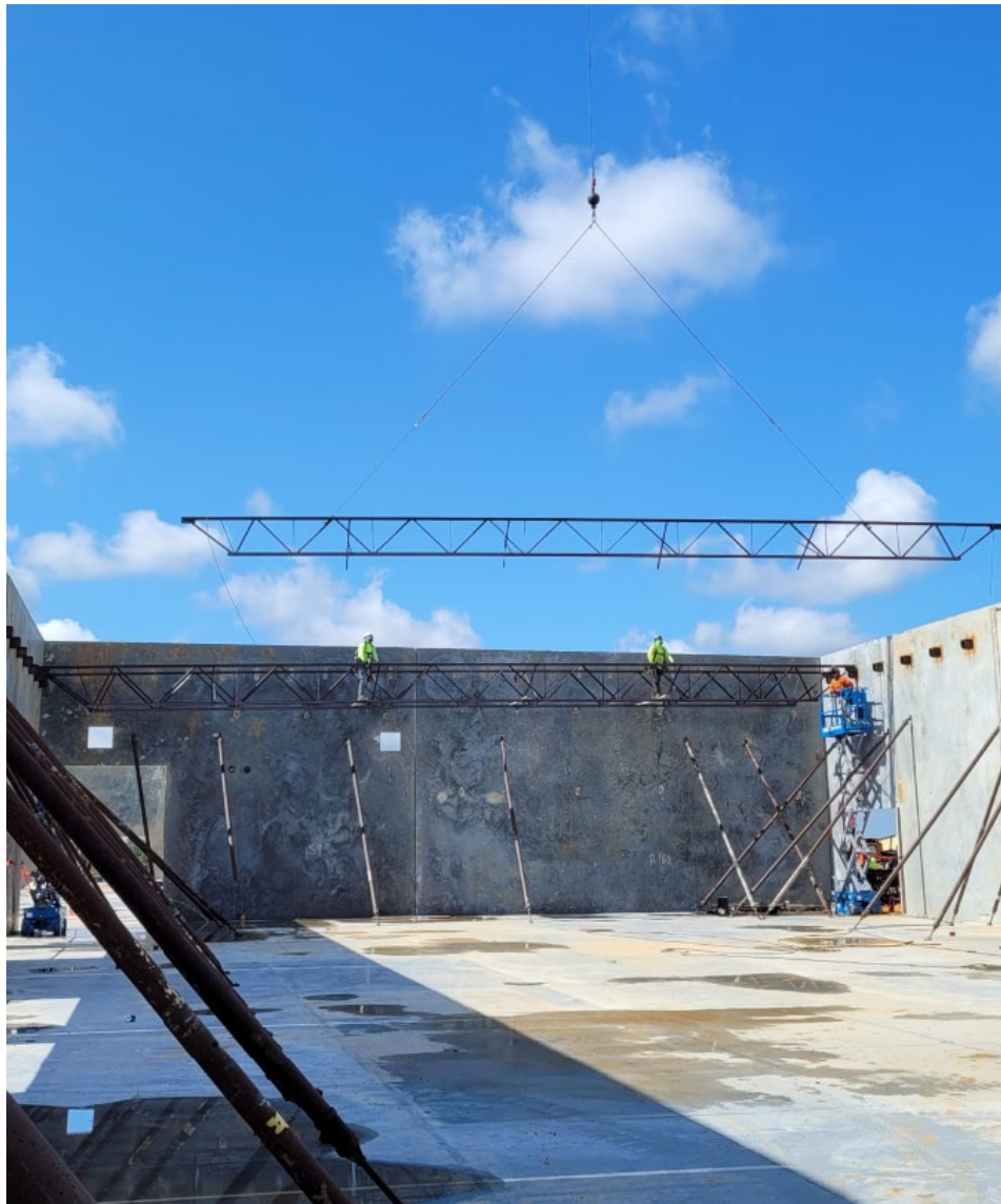
Above is placement of steel joists
