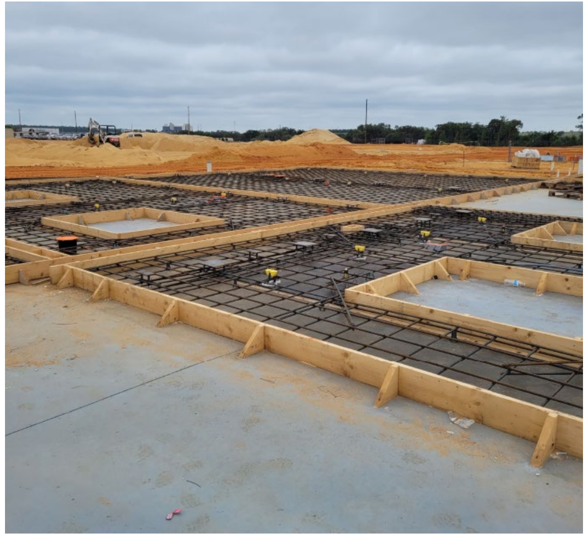
Above is tilt panel formwork with rebar, steel embed and blockout placements
