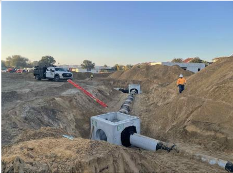
Installation of Civil (Storm) Underground Ongoing
