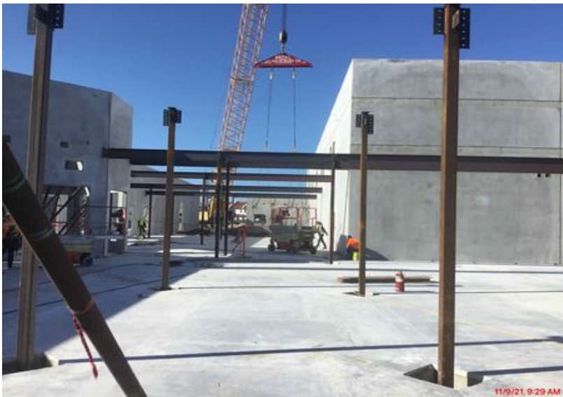
Setting of Structural Steel Columns and Beams
