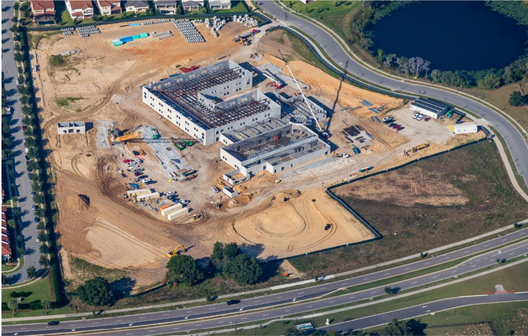
November 2021 – Site 114-E-W-4 : Erect Tilt Panels and Install Structural Steel
