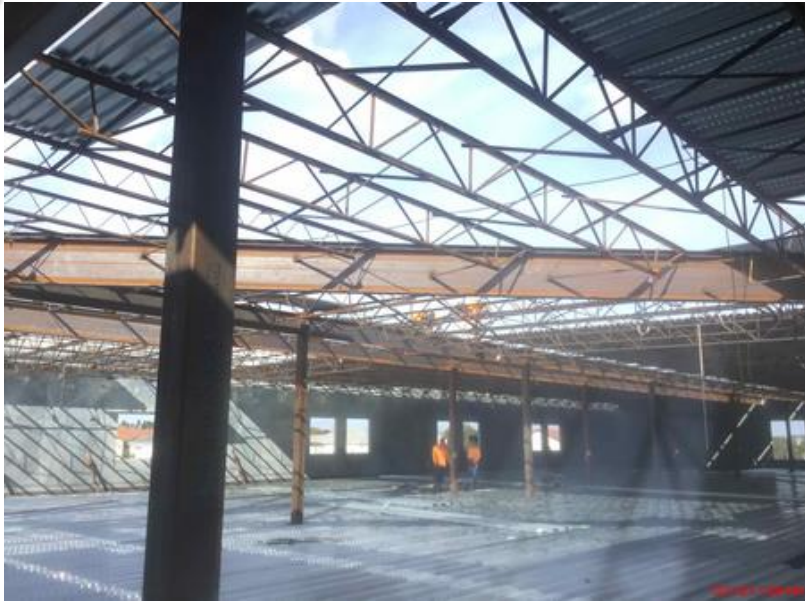
Metal Decking for Elevated Slab Complete and is ongoing for Roofing
