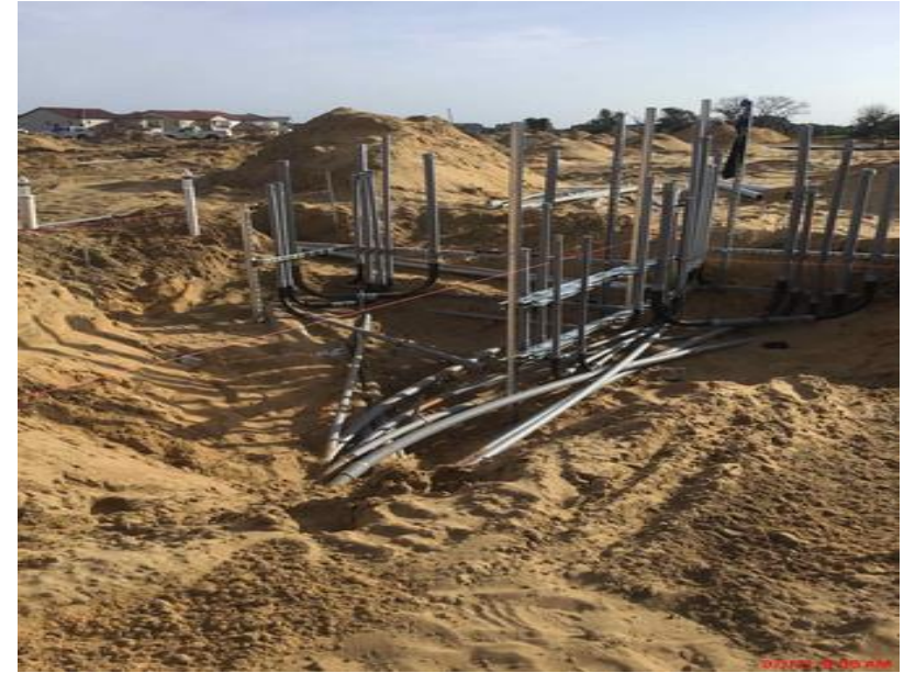
Electrical Underground Work at Interior Electric Room
