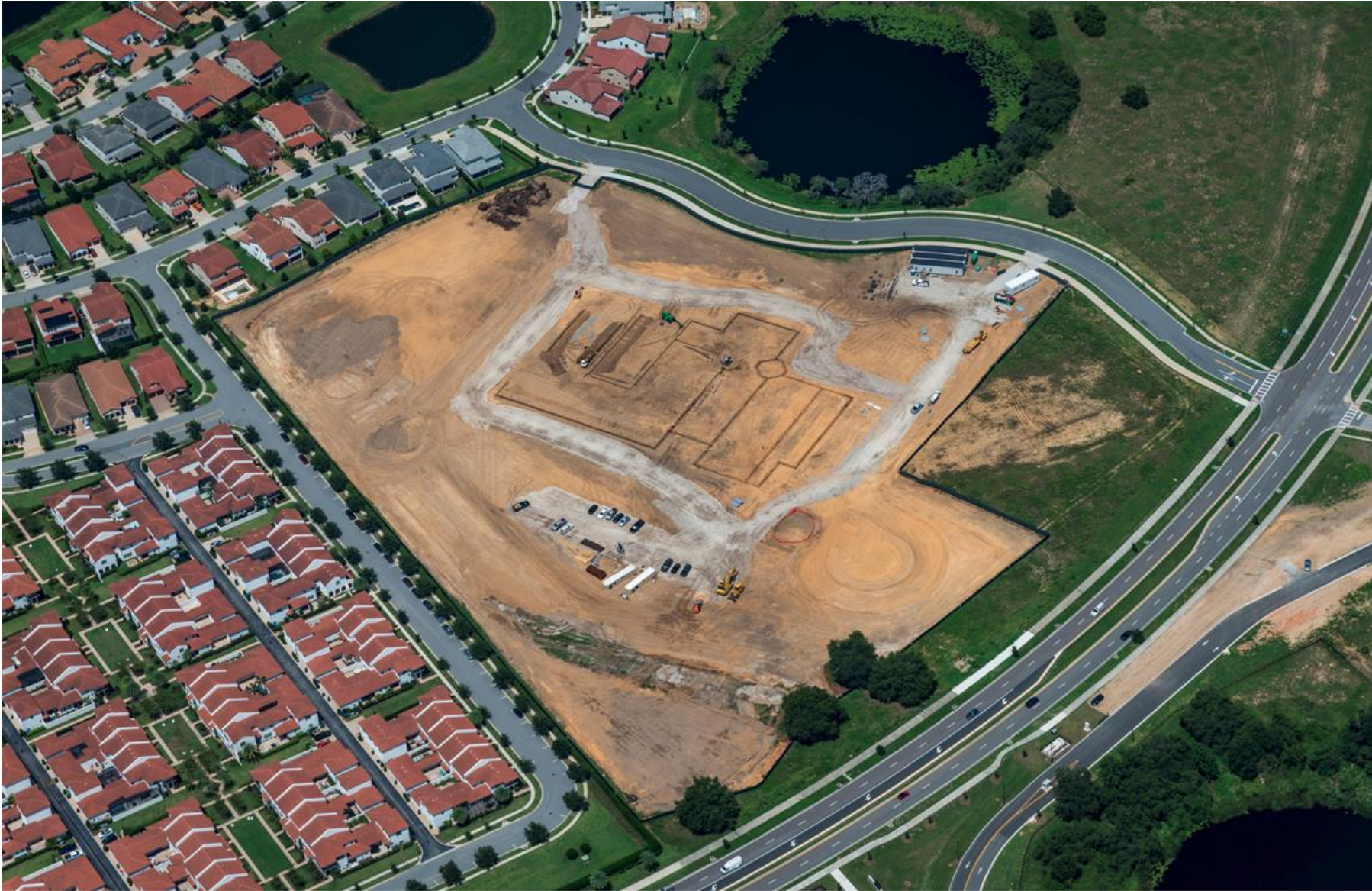
August 2021 – Site 114-E-W-4 : Project Access Roads, Jobsite Trailers and Foundations
