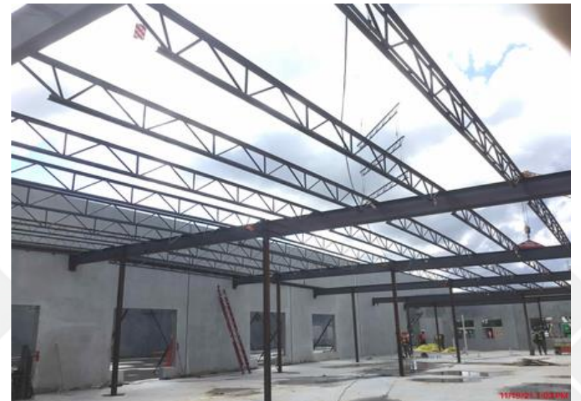
Setting of Structural Steel Joists
