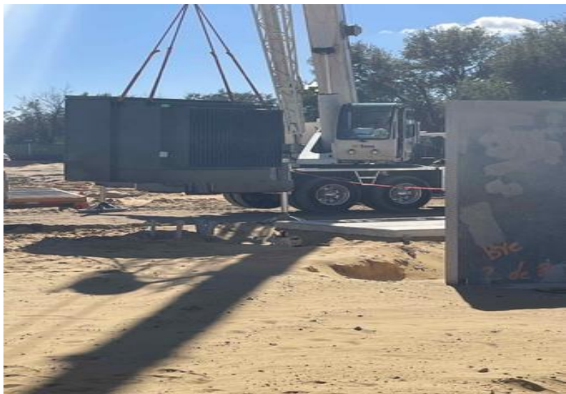
Main Electrical Transformer set and Energized
