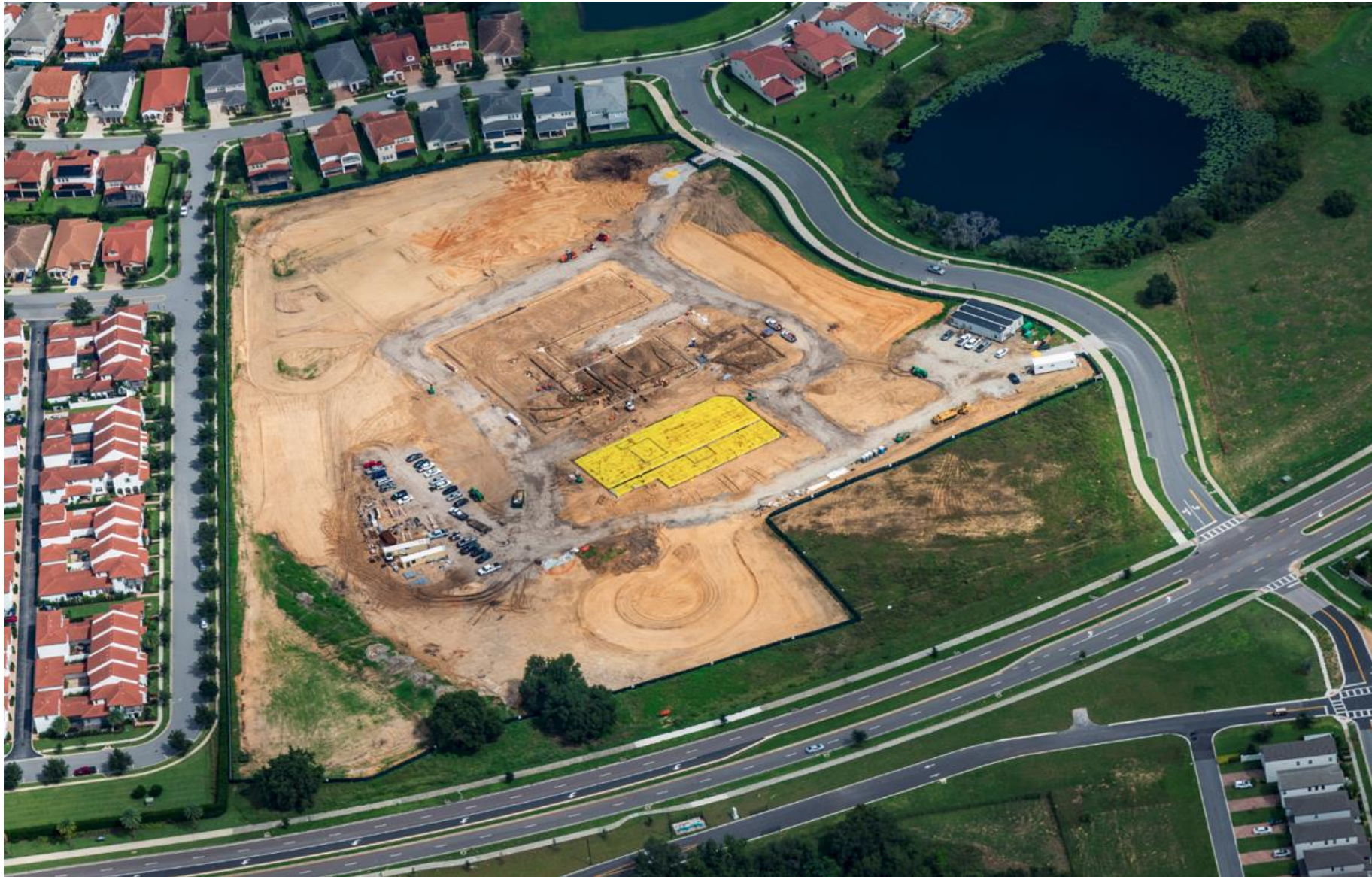
September 2021 – Site 114-E-W-4 : Mechanical, Electrical and Plumbing Underground and Slab-on-grade Pours
