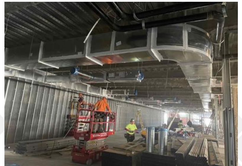
Above Ceiling Mechanical Duct being installed
