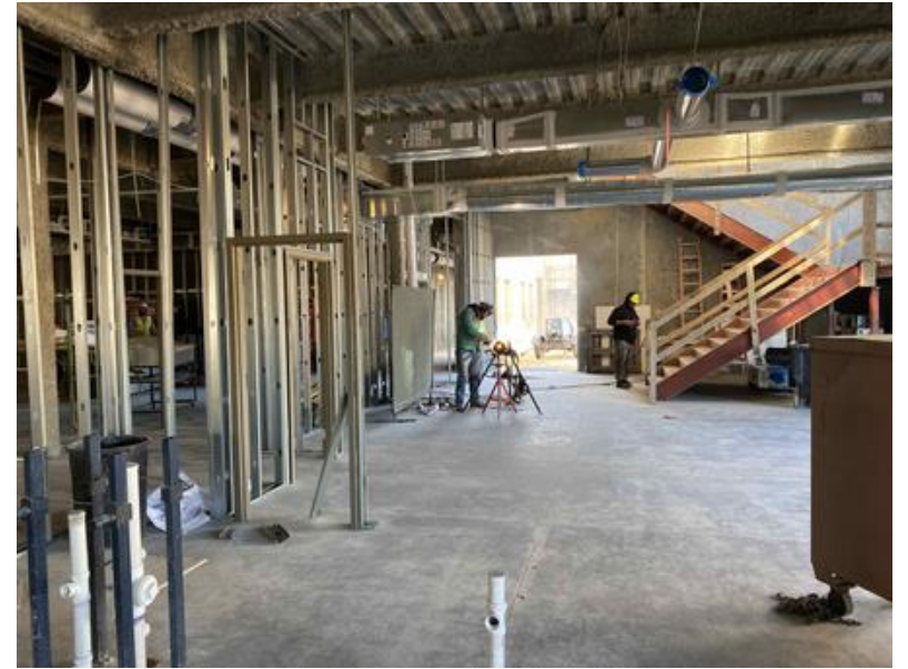
Metal Wall Framing including Mechanical, Electrical and Plumbing Rough is Underway
