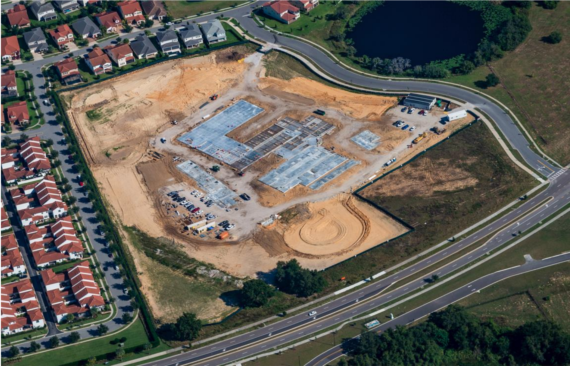
October 2021 – Site 114-E-W-4 : Forming Tilt Panels and Pouring Casting Beds
